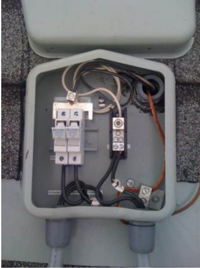
Left: Typical Residential Combiner, Right: Typical Commercial Combiner
