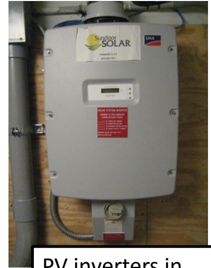
PV inverters in basements
