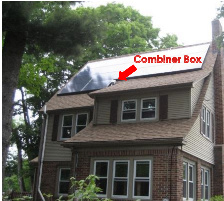
Residential Example: House containing PV on B and D sides.
