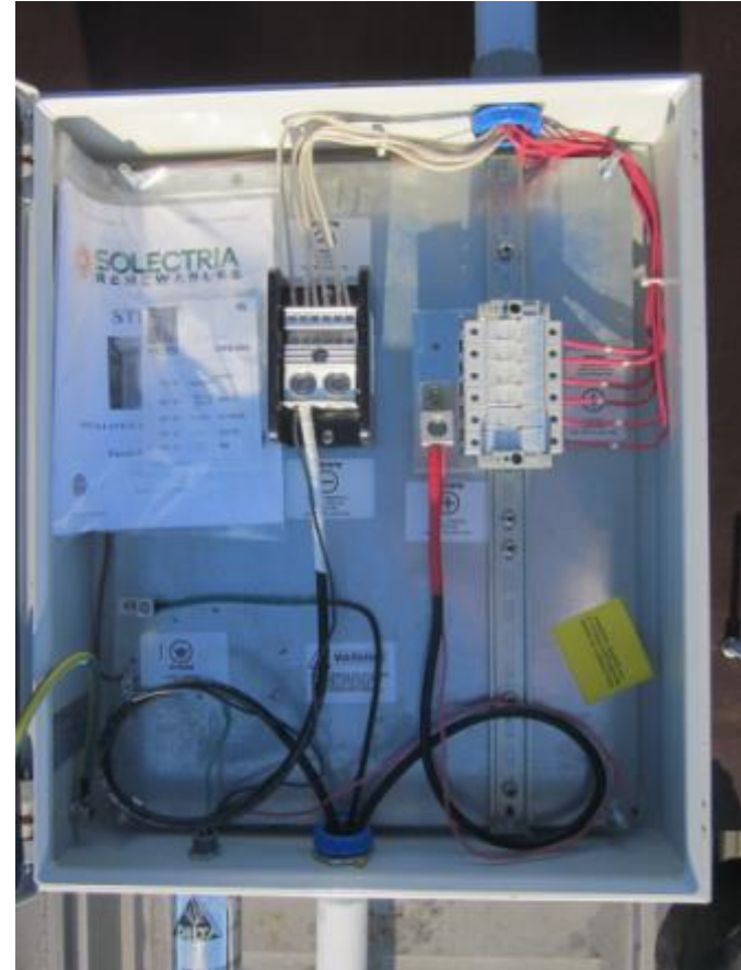
Left: Typical Residential Combiner, Right: Typical Commercial Combiner
