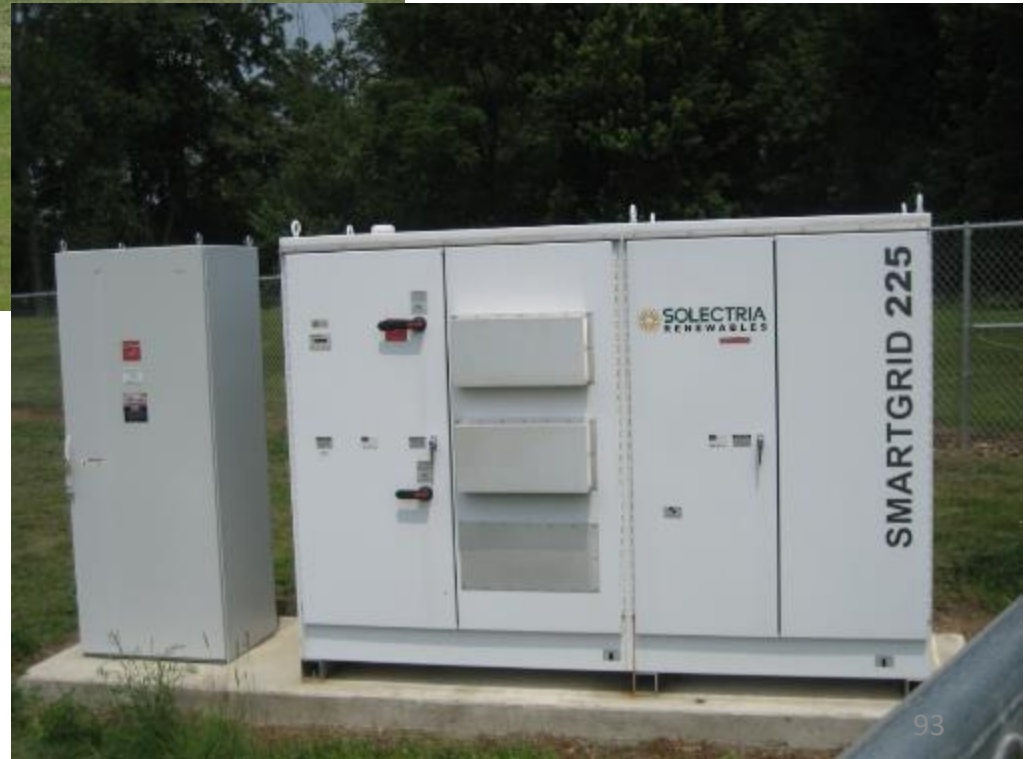
Example of ground-mount array, large Inverter and disconnects located remotely.
