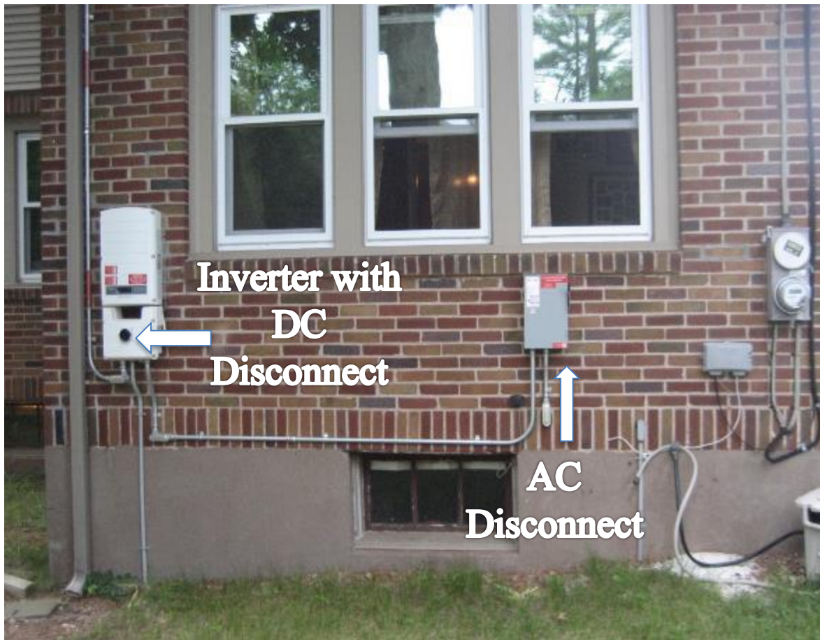
Residential Example: PV inverter and AC disconnect located on B side.
