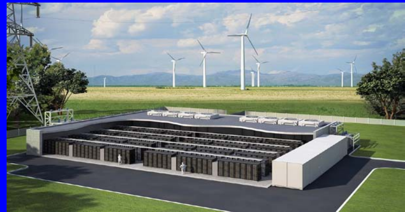
8MW / 4hr Li-Ion Storage for Wind smoothing - SoCal-Edison
