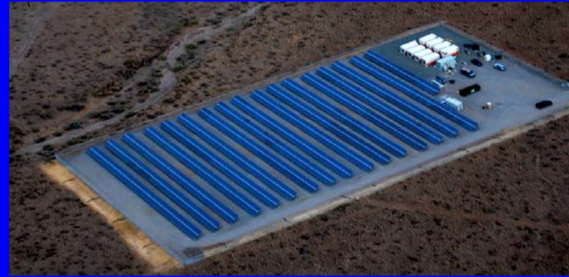
500kW, 2.5MWh PbC for smoothing 500kW PV - Public Service NM
